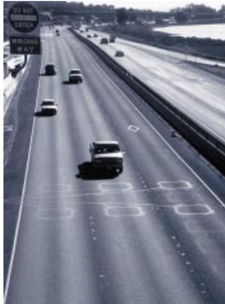
Above: Loop detectors in freeway. Above right: machine vision monitoring of traffic. Below right: CHP/Caltrans Transportation Management Center in Oakland, CA.
