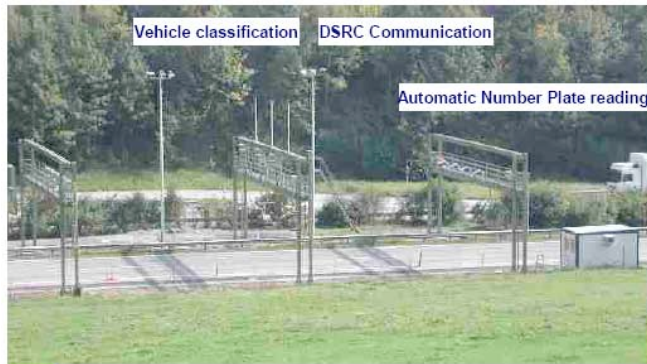
Figure 18: Swiss Control Gantries (Commission for Integrated Transport, 2006)
